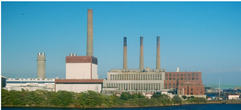
Mystic Generating Station
