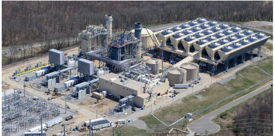
CPV Towantic Energy Center in early May, with construction nearly complete. | Competitive Power Ventures
